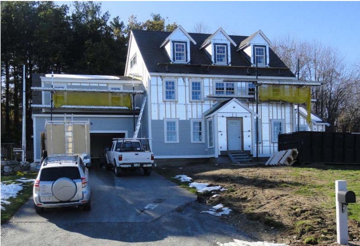
Westford DER: thermal package completed; exterior trim & siding being installed
