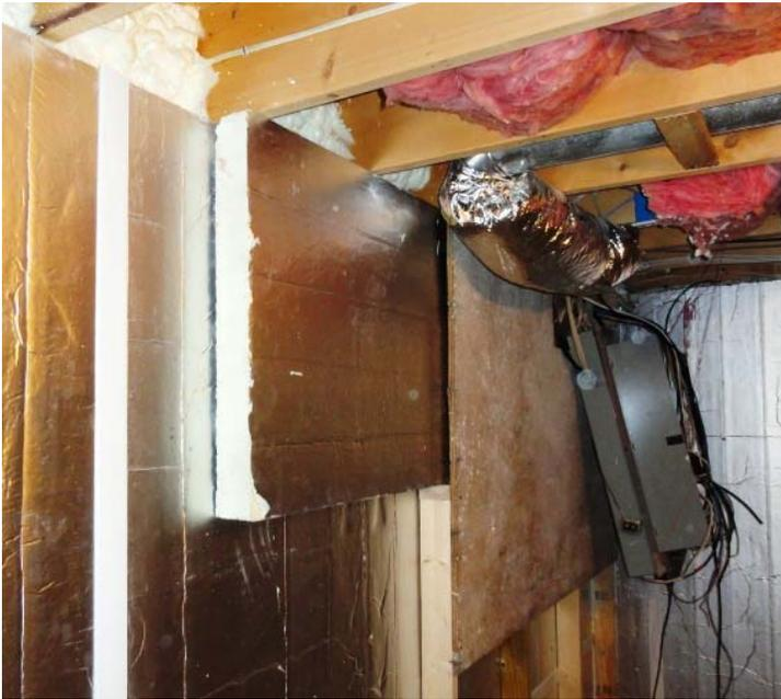
Westford DER: Basement Insulation being installed
